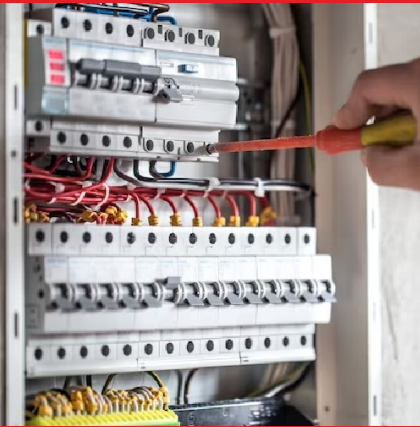
EXECUTION OF ALL ELECTRICAL WORKS
