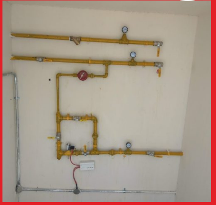
WIRING & EXTENDING COOKING GAS PIPES IN RESIDENTIAL FACILITY & VILLAS
